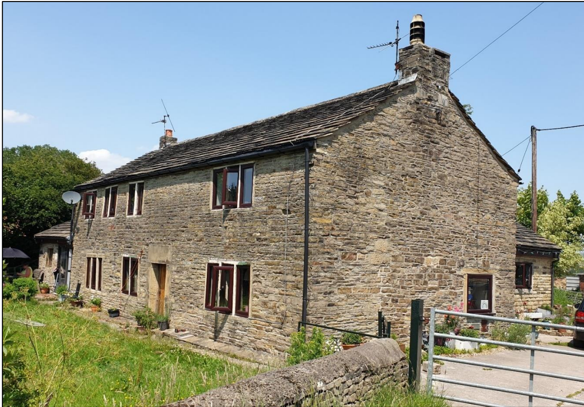
Plate 12 4 Greenside Farmhouse, mid-17th century in date. The 19 th century hatting workshop can be seen to the left
