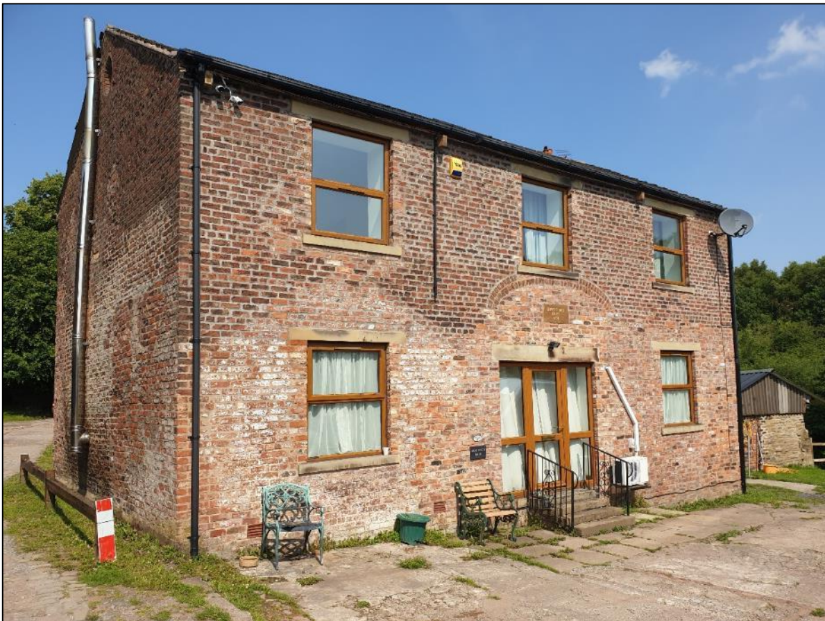
Plate 18 The former barn at Brookfold Farm
