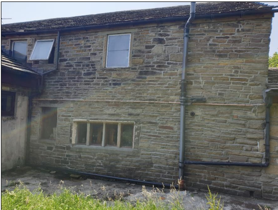
Plate 13 The ground floor range of mullioned windows is believed to be original to the house and 17th century in date
