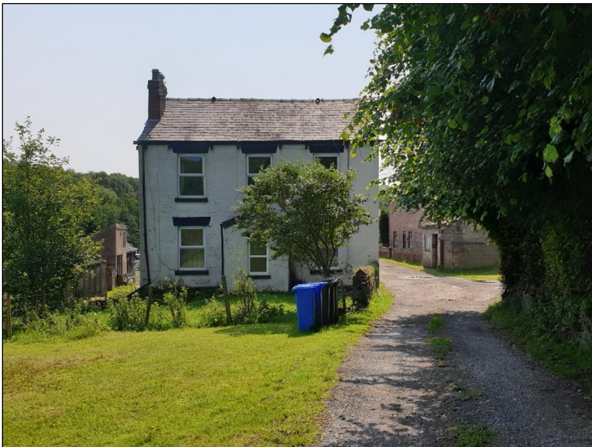
Plate 20 Early 19th century farmhouse at Brookfold Farm
